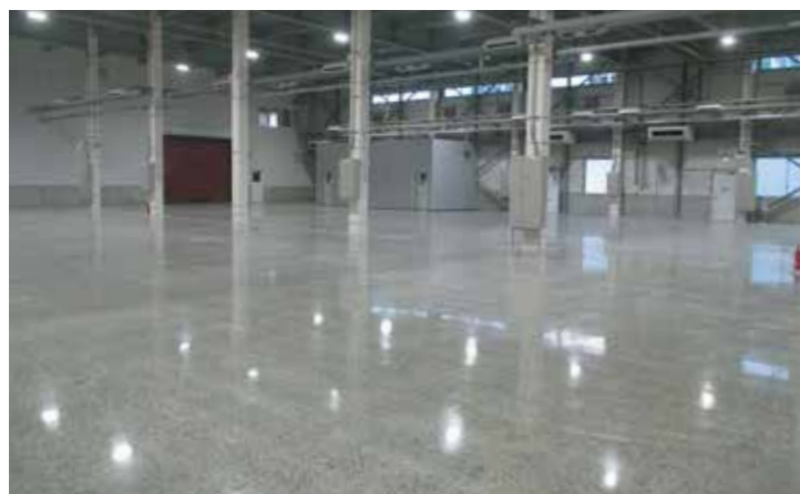
New plant at Oharu Works
