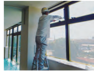
Thermal barrier paint being applied to window glass
