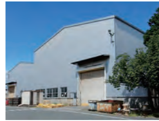
Factory with heat shielding and insulation measures on exterior walls
